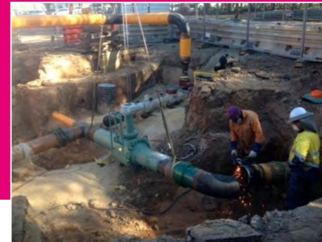
Medium and high-pressure gas mains were located and diversions identified in conjunction with National Grid Gas. Diversions were planned for times of low gas demand, mainly in the summer, and when mains could be emptied or supplies routed via other mains, or when this was not possible stopple pits and hot tapping methods were used.
